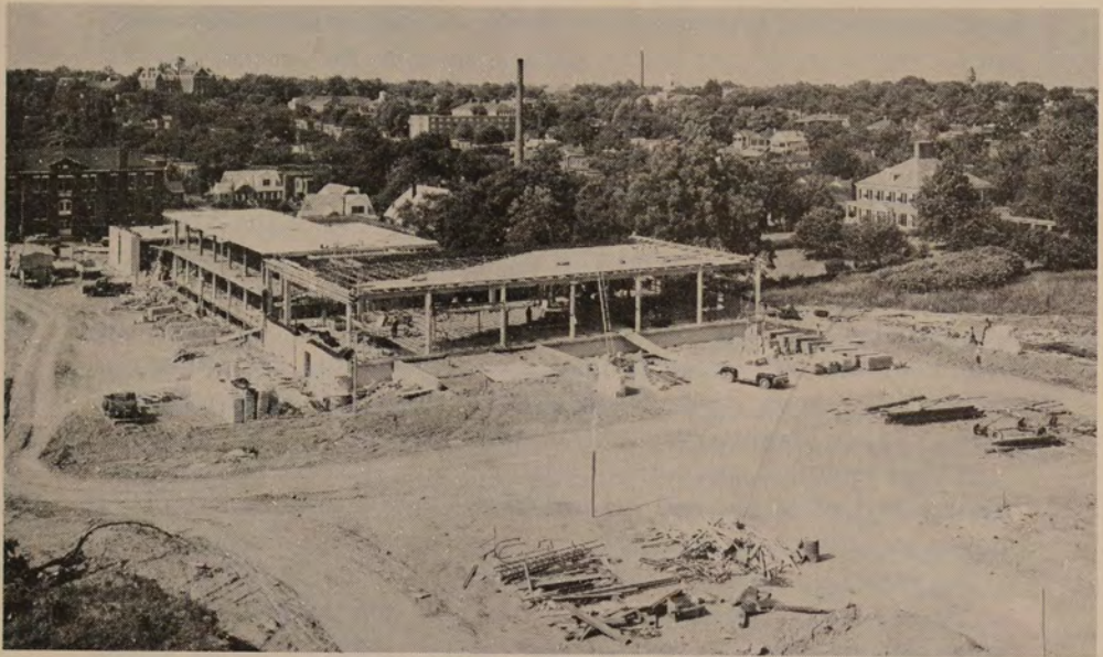
ITC Under Construction
