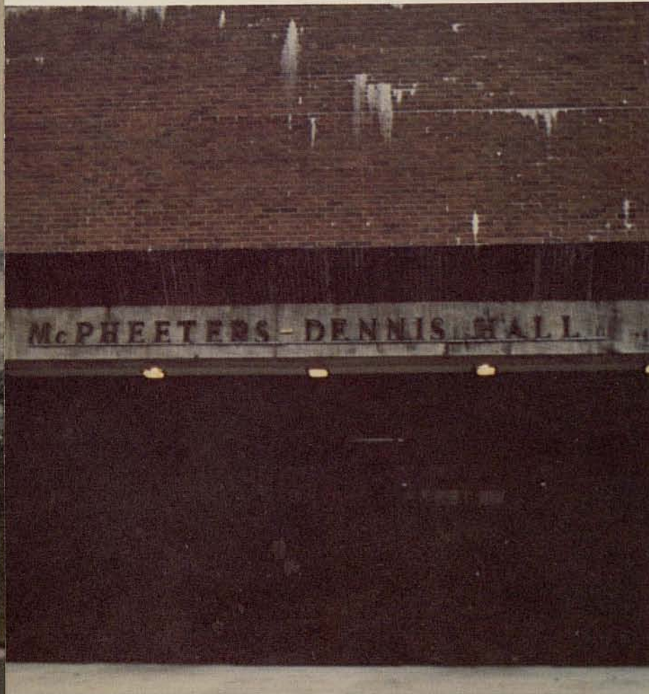
Above: WCLK, Marquis L. Harris library, science, math and Mass Communication courses and departments resided in McPheeters-Dennis Hall. Right: Haven Warren Administration Building is shown in the background of the fountain which depicts similar meaning and memories to the Clark College family.
