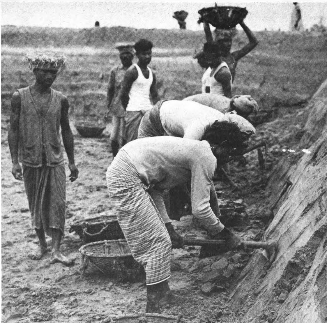
Food For Work Scheme. By the end of March 1985, hundreds of laborers will have completed a great earth embankment in Western Sylhet, which will protect 30,000 acres from early floods. Crops will then be able to be grown on this previously fallow land.
